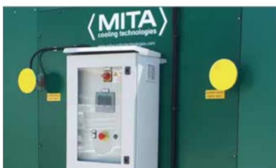
MITA Control System: integrated control system equipped with inverter.
