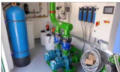
Technical room for housing control equipment: pumps, inverters, control panel, water treatment systems.
