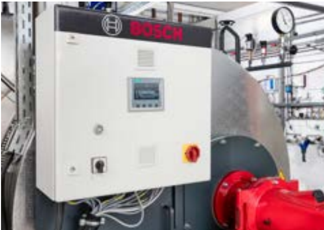
Compact steam boiler control CSC
