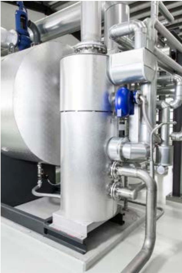
Expansion, heat recovery and blow-down module EHB
